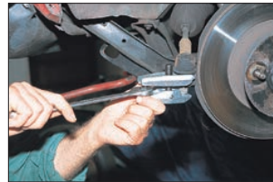
A puller is used to pry off the tie rod ends.
